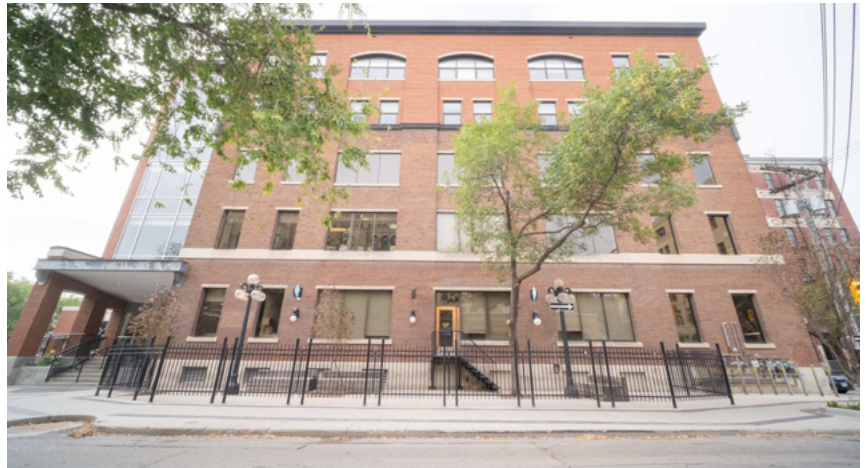
The exterior of the building housing MCC Manitoba's new offices at 140 Bannatyne Avenue, Winnipeg. The café Sam's Place, where MCC Manitoba's youth program takes place, is located on the main floor. MCC photo/Michael Veith
